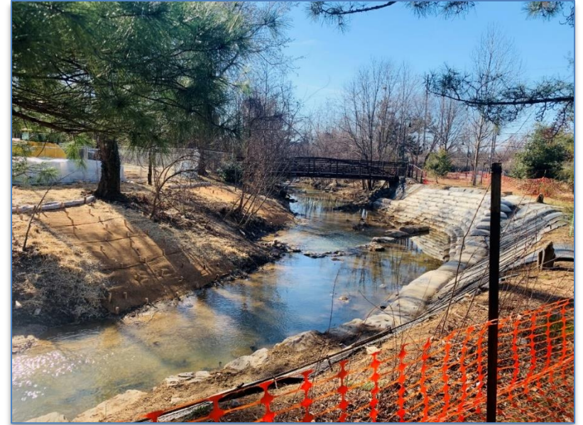
Emergency stream bank repair, DC
