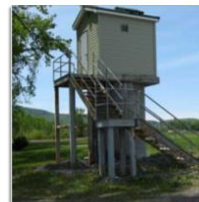
Wellhead Elevated above BFE (U.S. EPA)
