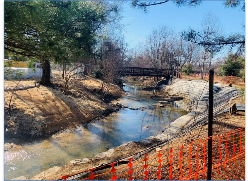
Emergency stream bank repair, DC
