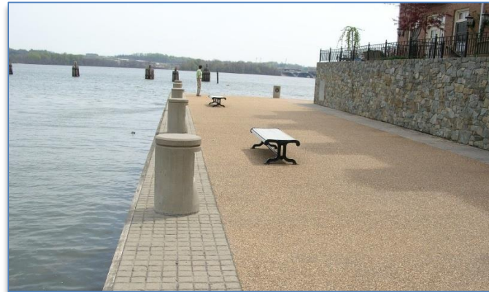
Windmill Hill Bulkhead, Alexandria, VA
