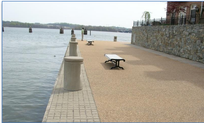
Windmill Hill Bulkhead, Alexandria, VA
